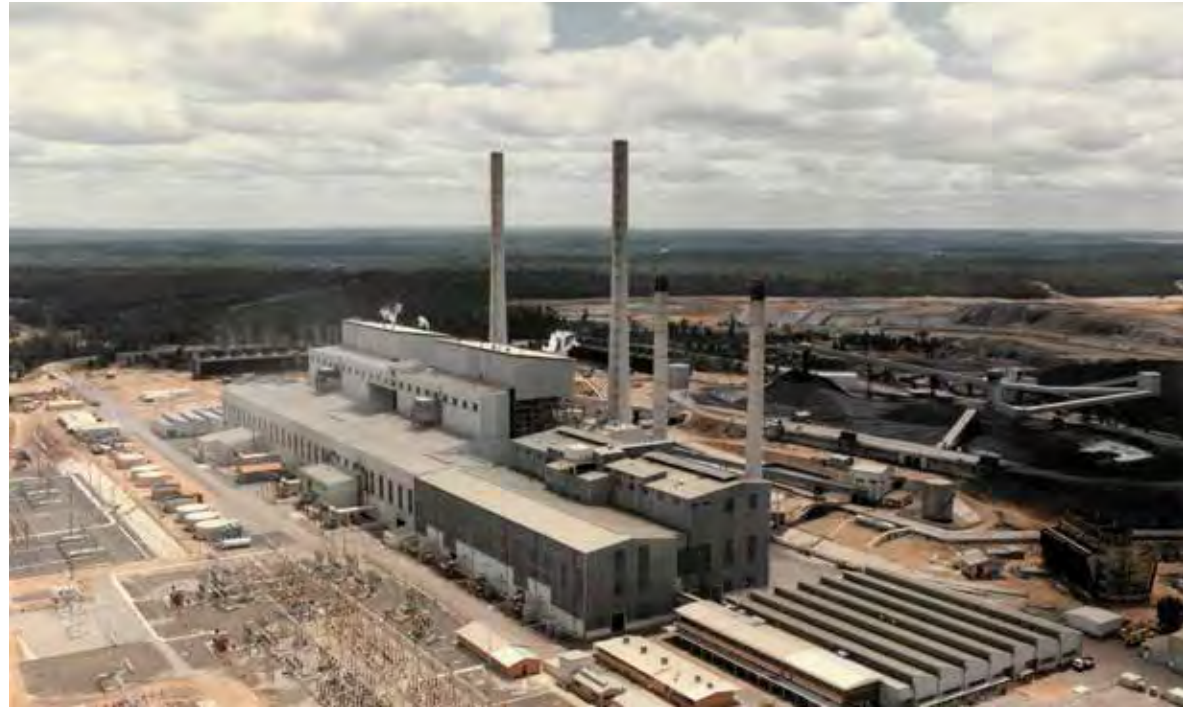
Muja Power Station
