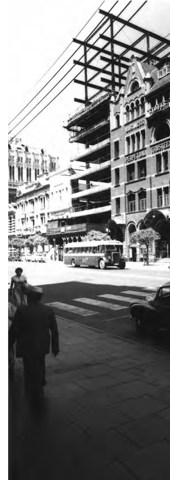
Construction of the National Mutual Building
