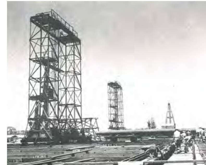
Construction of the Narrows Bridge
